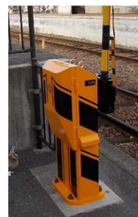
踏切遮断機更新
