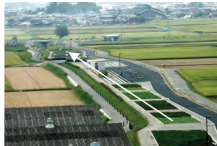
Fig. 4-7-4 Project to purify wastewater discharged from urban land (Purification of wastewater from urban land such as residential areas and roads by means such as capturing wastewater, sedimentation, plants and soil)
