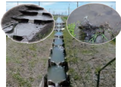
Fig. 3-13-4 Weir type fishway where crucian carp and catfish swim upstream
