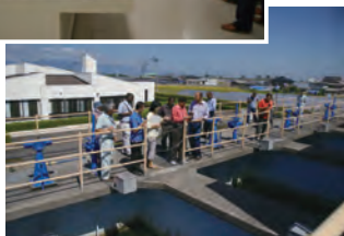
Kitayamada Purification Plant
