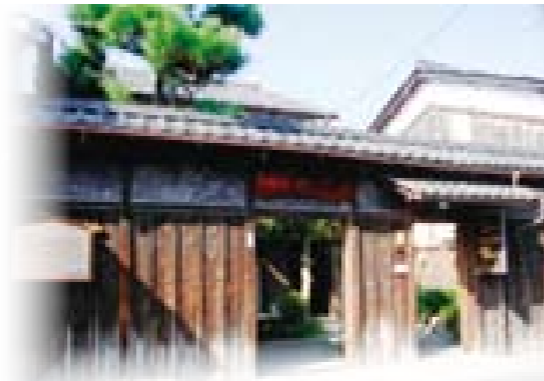
NO = MA 建物外観
