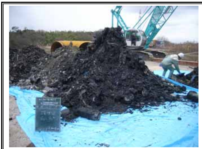
掘削廃棄物土 (GL-6.00 ~ -9.00m)
