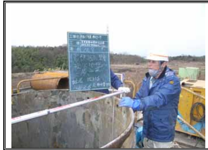
掘削深度確認(GL-14.20m)
