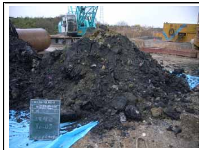
掘削廃棄物土 (GL-9.00 ~ -12.30m)
