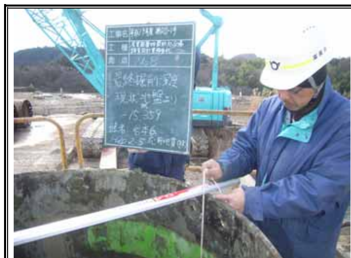
掘削深度確認 (GL-15.35m)
